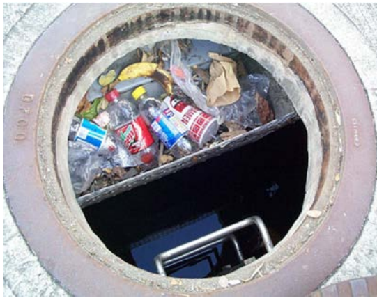
Catch Basin Insert from the City's "Efficiency of Storm Drain Filters in Removing Pollutants from Urban Road Runoff"
