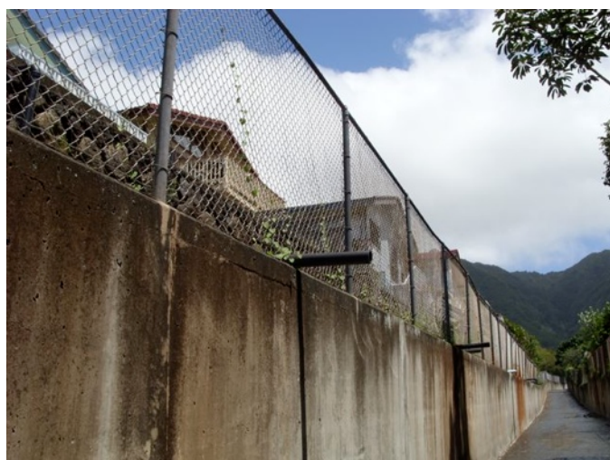
Figure 13: Almost all houses along Kuliouou channel in the upper reaches have pipes connected to the stream channel. Stains and biofilms are obvious along the bank walls, possibly suggesting high nutrient input or organic matter.
