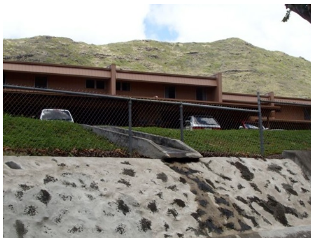
Figure 14: Concrete drainage connected to Kuliouou channel from parking lot of Haleloa I, a multifamily complex. Decreases filtration of runoff before entering channel and drains a parking lot directly (hotspot).
