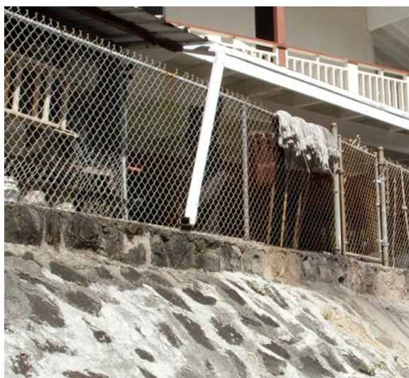
Figure 12: Example of rooftop downspout connected to stream channel from residence along Kuliouou channel.
