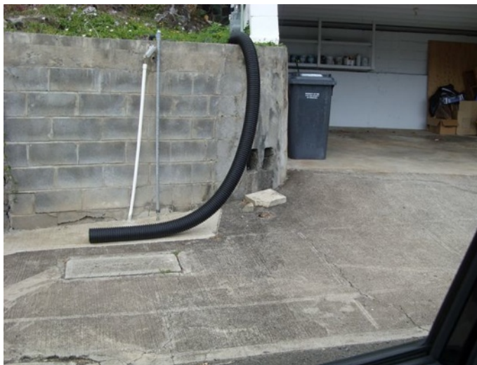
Figure 8: Pipe running from residence directly to sidewalk, a very common practice in Wailupe neighborhoods (Aina Haina). Pipe is connected to impervious surface and decreases filtration of runoff before entering the stream channel.
