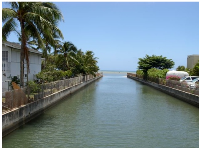
Figure 10: View of Kuliouou channel near Kuliouou Beach Park. Kuliouou is a typical drainage in Maunaloa Bay area, as it has been straightened and lined with concrete in its entirety.
