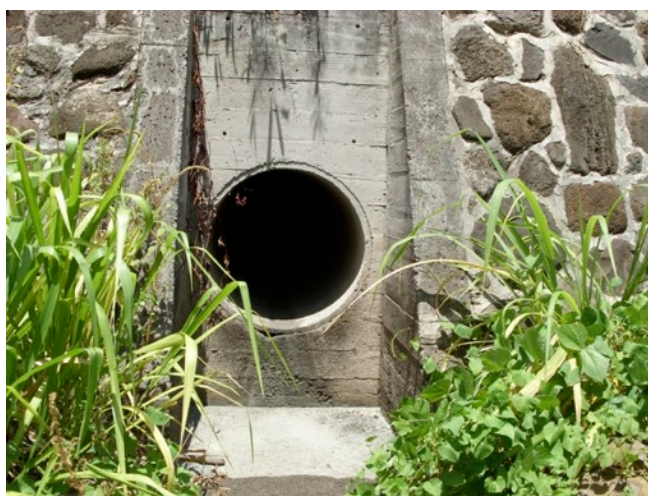
Figure 6: Typical storm water outfall observed along Wailupe stream, roughly 1 m in diameter. Outfalls were clean and usually few of plant debris.
