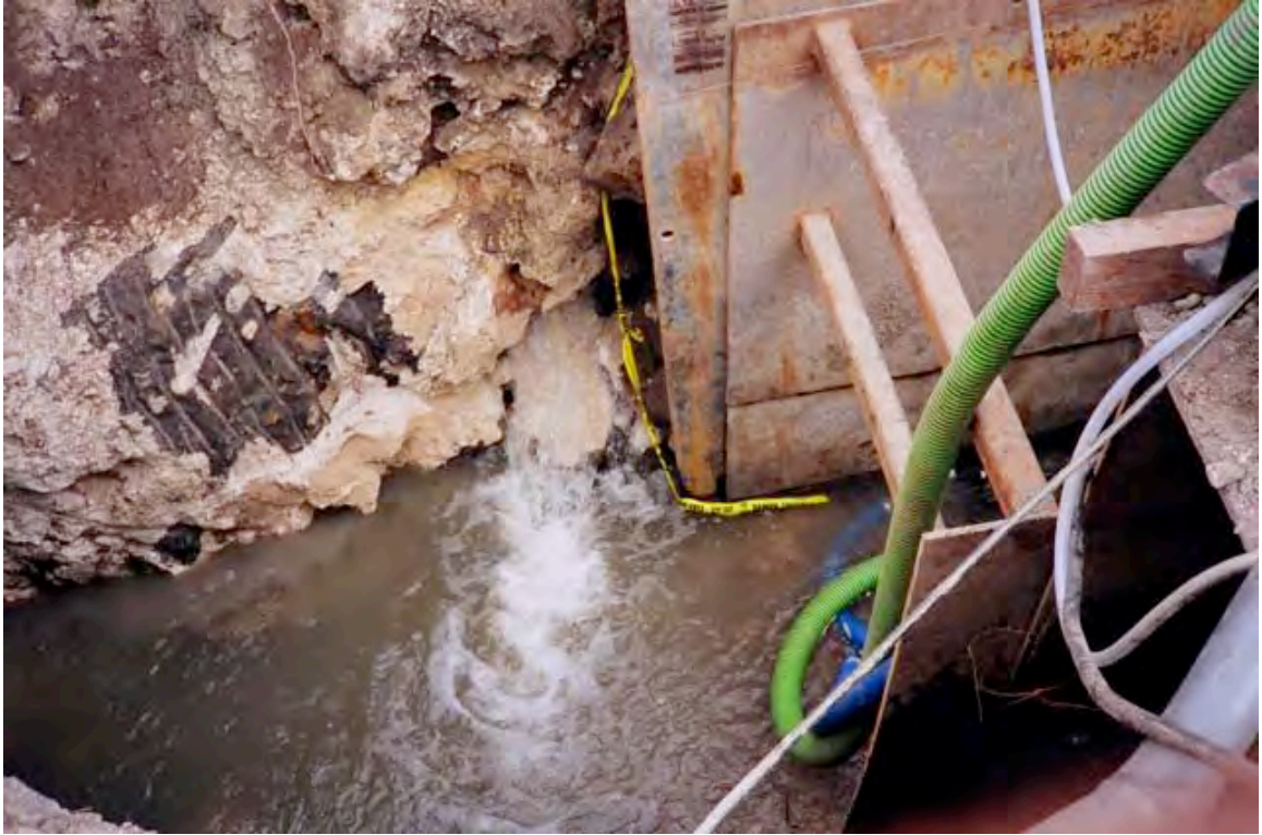
Figure 5. Water flowing out of probable broken lava tube conduit during the Kalaniana'ole Highway widening project, ca. 1993. Photo: T. Hara, courtesy MFHC.
