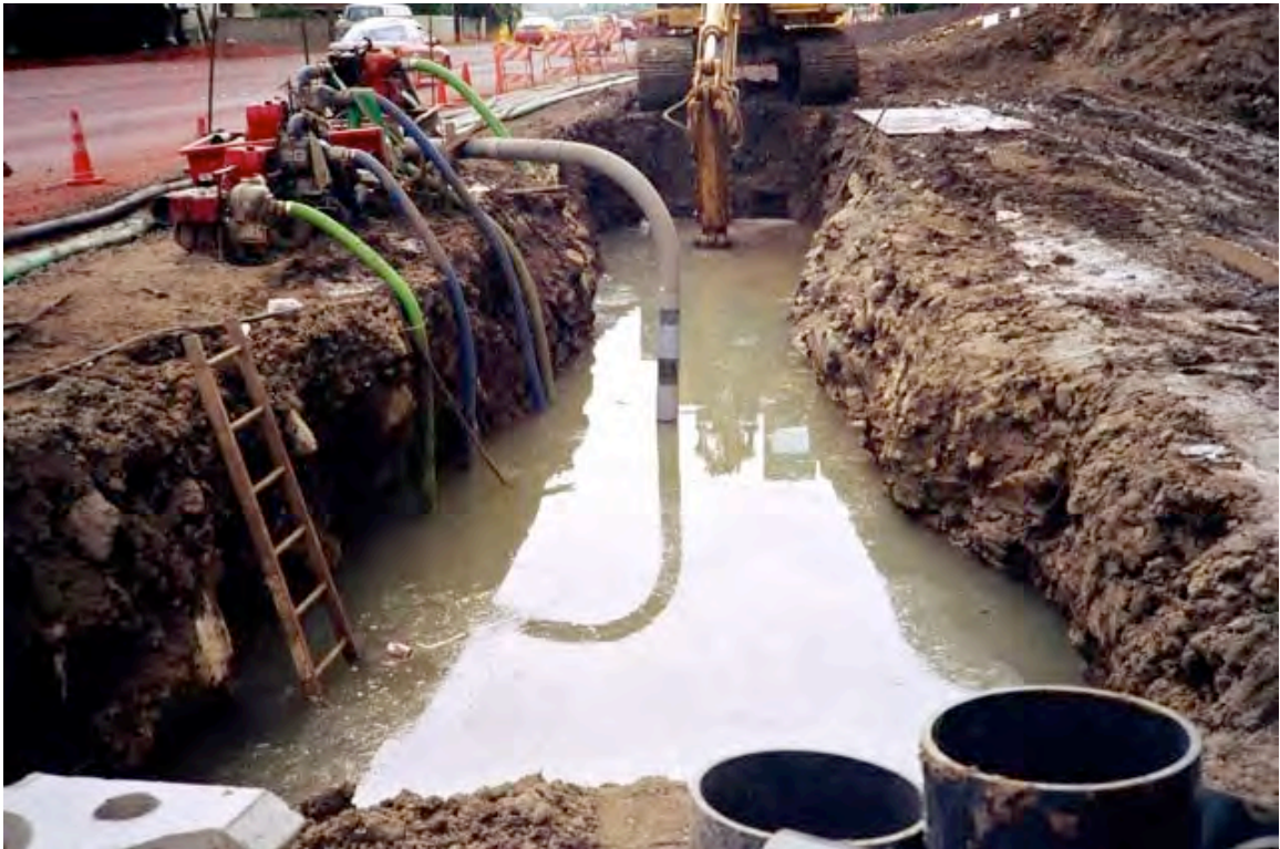
Figure 6. Water being pumped from flooded construction site landward of the Lucas Spring Study Site, ca. 1993. Photo: T. Hara, courtesy MFHC.
