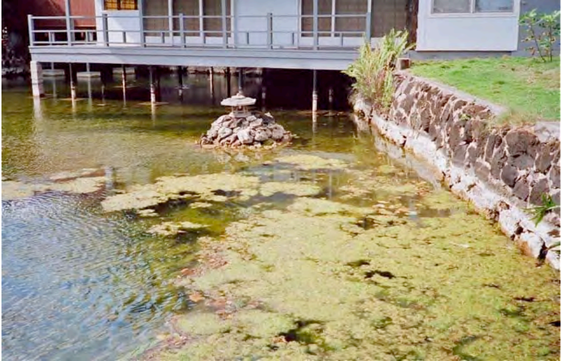
Figure 8. View of Lucas Spring after the freshwater conduit was severed and beginning to deteriorate, ca. 1993. Photo: T. Hara courtesy of MFHC.
