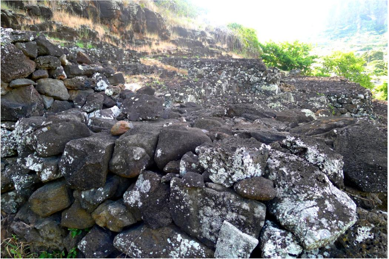
The western wall of Pahua Heiau, Maunaloa, O'ahu. Source: OHA 2014.
